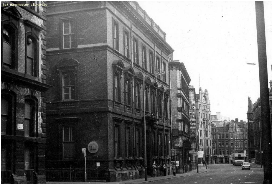
Original College of Commerce building [1973]
