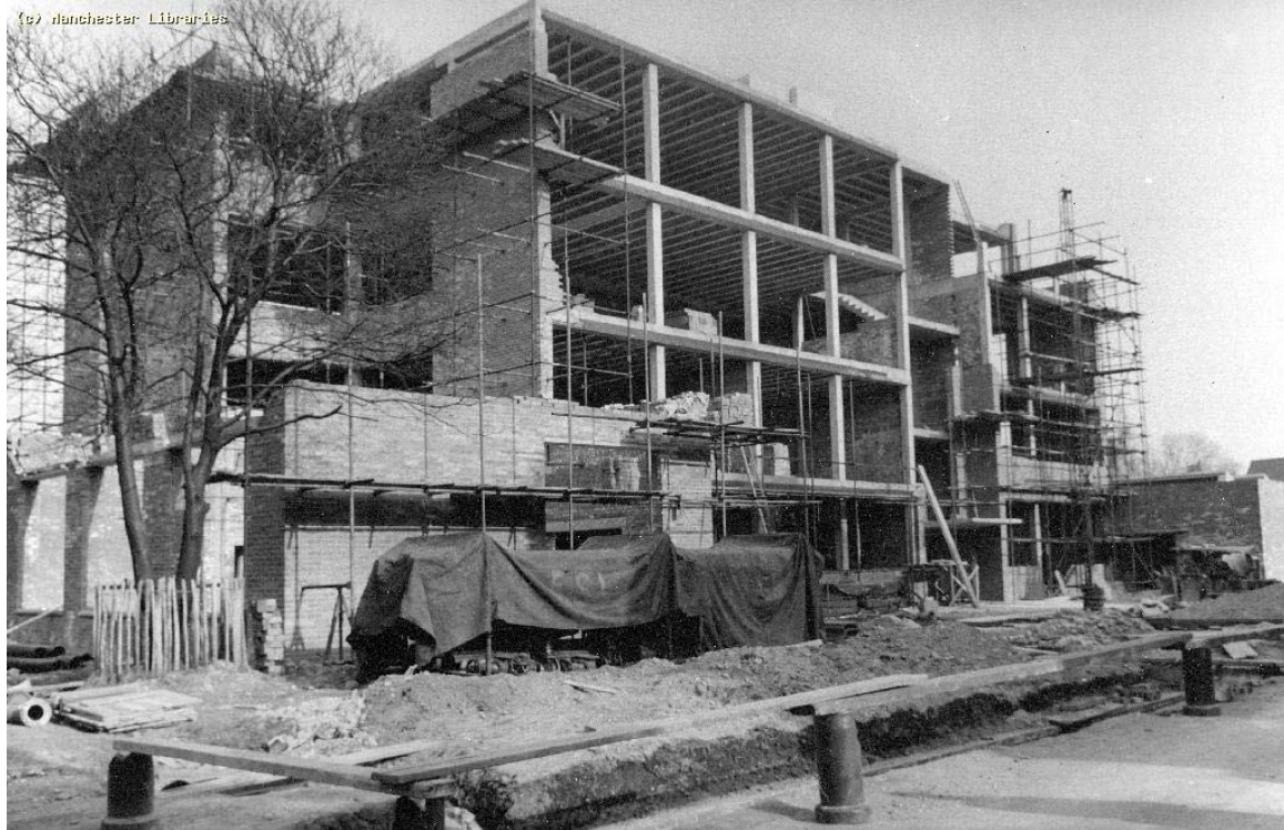
Didsbury College Campus under redevelopment in the 1960s
